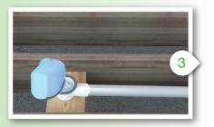
Cut a piece of plywood to support the drain for drain body, this should be 10mm higher than waste pipe. Connect the drain body to the waste pipe with solvent weld in the usual way. (Always check for leaks before final installation of shower tray).
