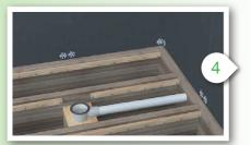
Fix a batten below the top of the joists.
